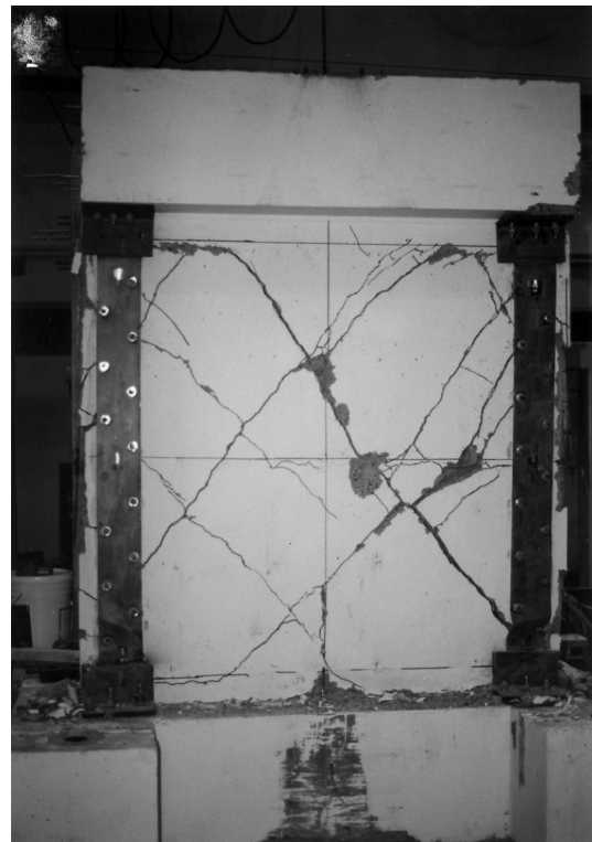
FIG. 11. Cracking Pattern of Wall 11RP
